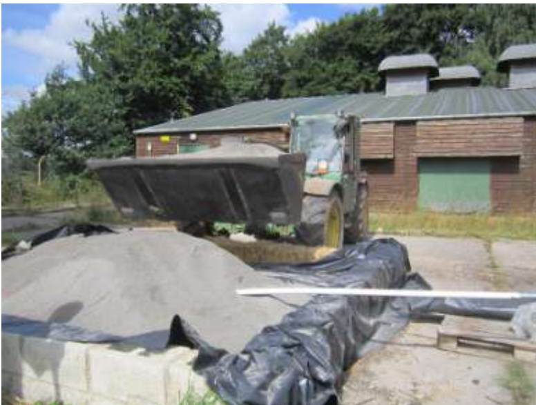
Figure 2.4 Construction of the PS storage heaps
