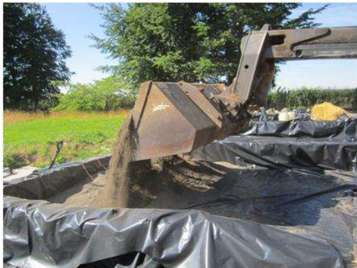
Figure 0-3. Construction of the PLA storage heaps
