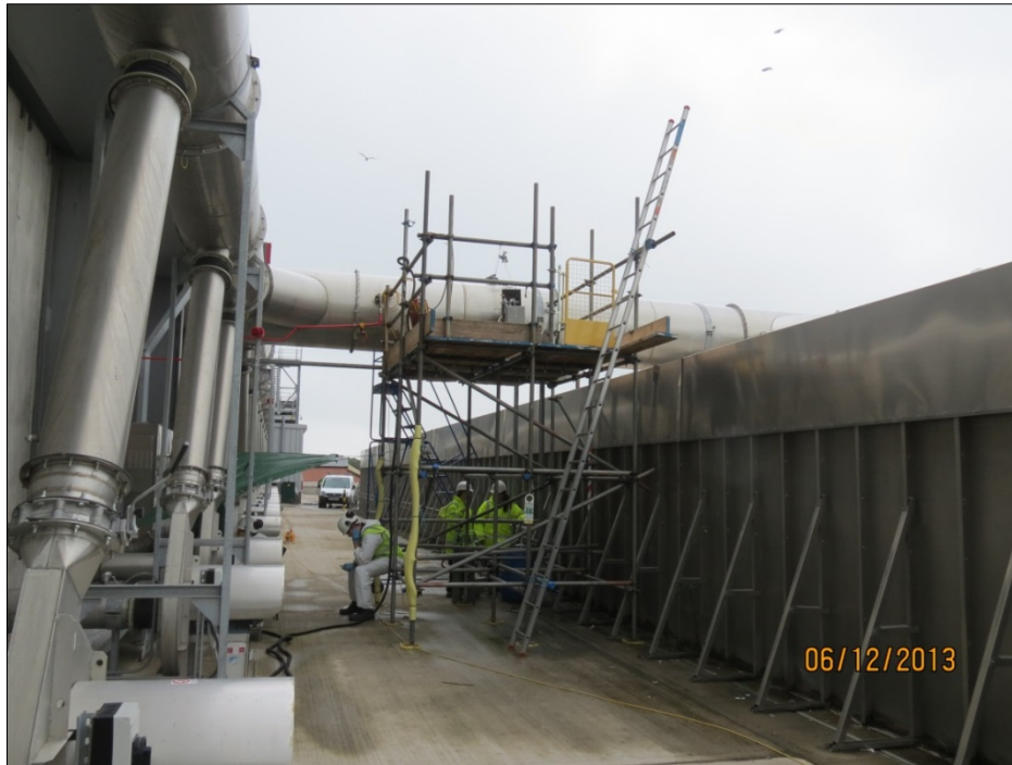
Plate 2 Sampling port in the inlet duct to the biofilter at Site UOL01
