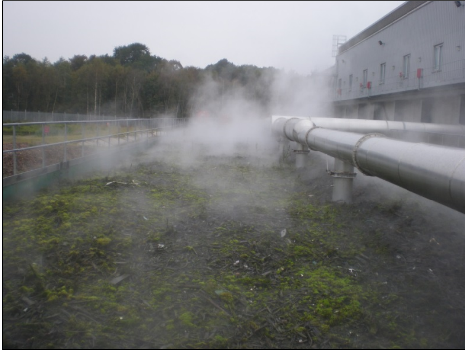
Plate 4 The open biofilter at UOL05, showing the surface of the biofilter and the arrangement of the inlet duct.
